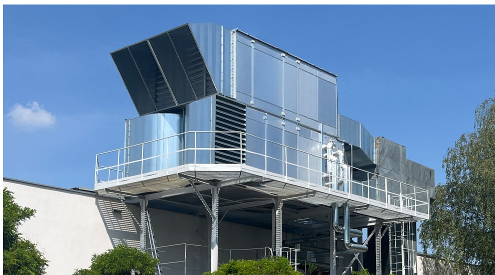
Ventilation system upgrade investment at the Poznan factory in Poland.
